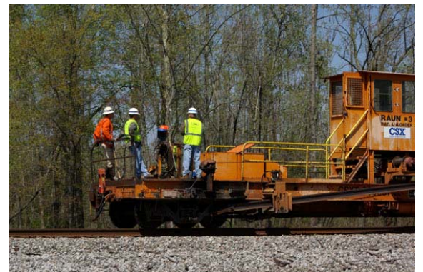
CSX ribbon rail train in siding at Romney
